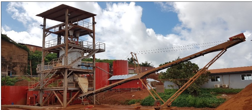
Figure 16. Processing plant fresh tailings. Vertical process arrangement: 2 hydrocyclones on top, static flow to the hydrosizer AKA-SIZER and direct discharge of the valuable fraction to the dewatering screen below.
